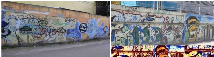
Figure 3. Illegal Graffiti in Medan Timur Figure 4. Illegal Graffiti in Medan Helvetia
